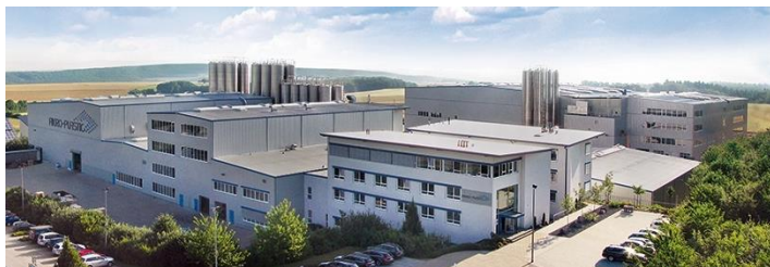
Production plant Niederzissen
